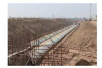
FRP pipe with sand Specification: DN10~DN3000mm、PN0.1~2.5MPa、 SN1250~SN20000N/m2
