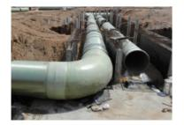
FRP pipe Specification: DN50~DN4000mm、PN0.1~3.2MPa、 SN1250~SN20000N/m2
